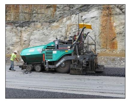
Mixtures placed with Wirtgen Vogele Rubber Tired Paver
