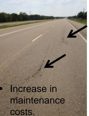
Thermal streaks; areas with increased potential for longitudinal cracking.
