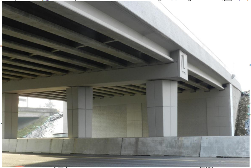
Pier Elevation - Segmental Columns and Precast Bent Cap
