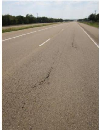
• Effect of reduced compaction because of lower mat temperatures or inadequate rolling.
