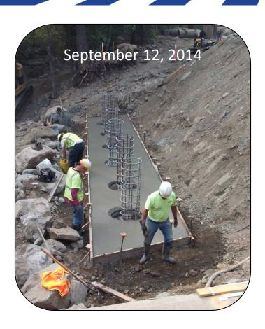
4 sac slurry for abutment bearing pad proved an effective leveling pad.
