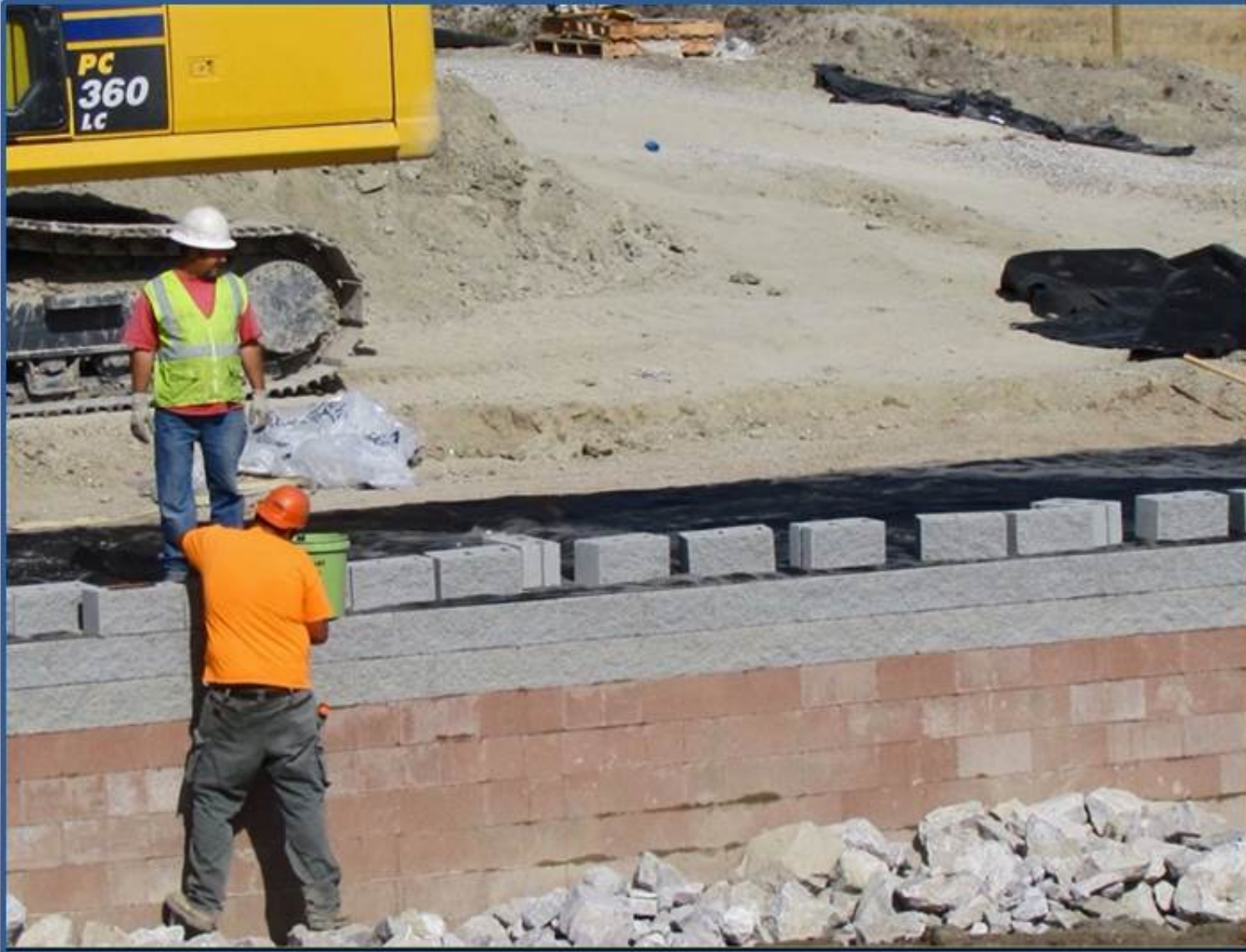
Geotextile Reinforced Soil
