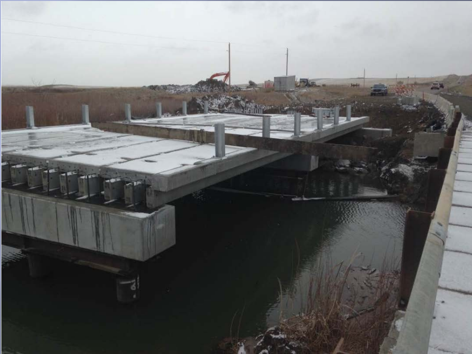
Prefabricated Bridge Element System – Tri Deck Beams
