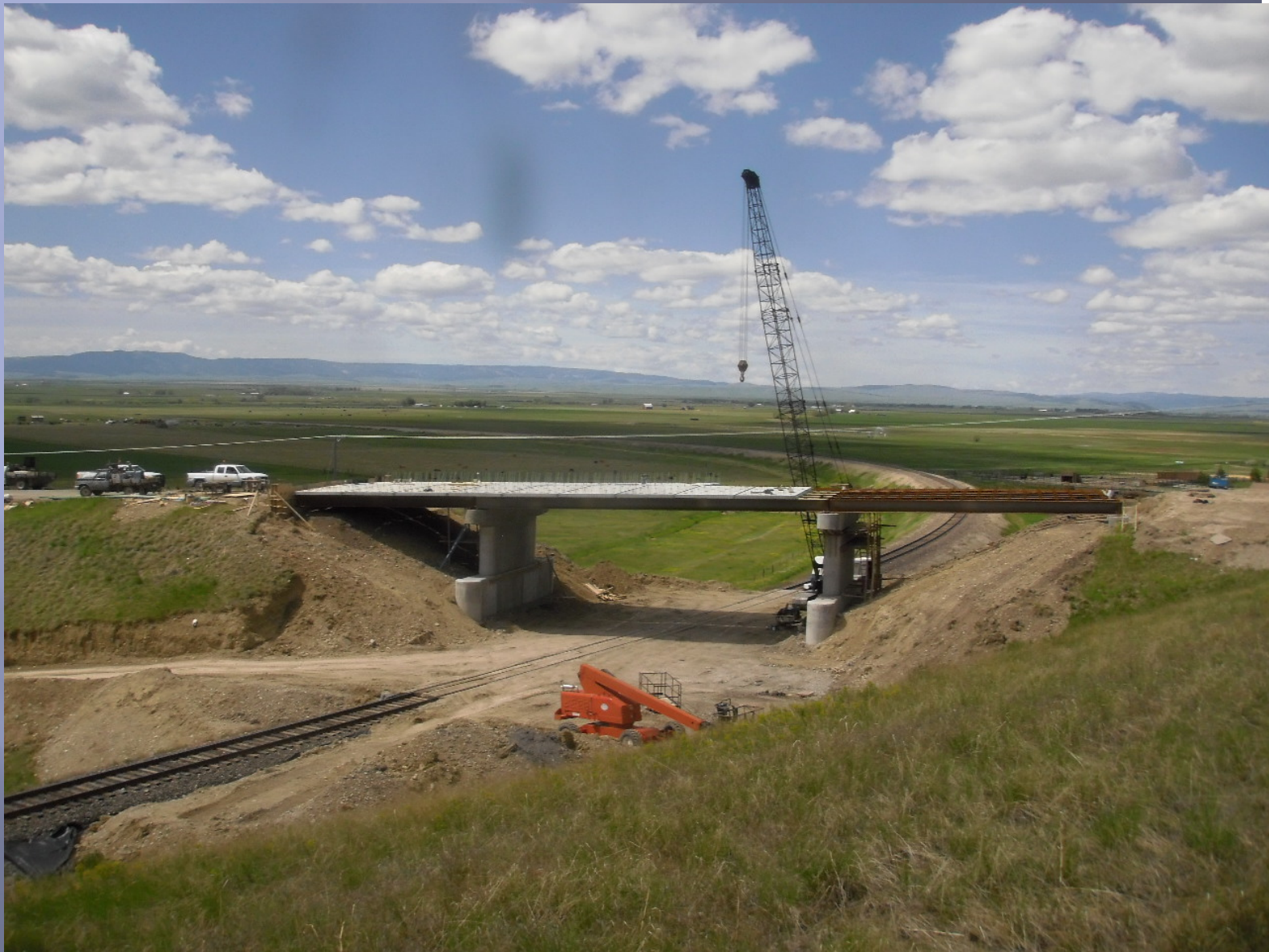
Longitudinal Concrete Deck Panels on Steel Girders
