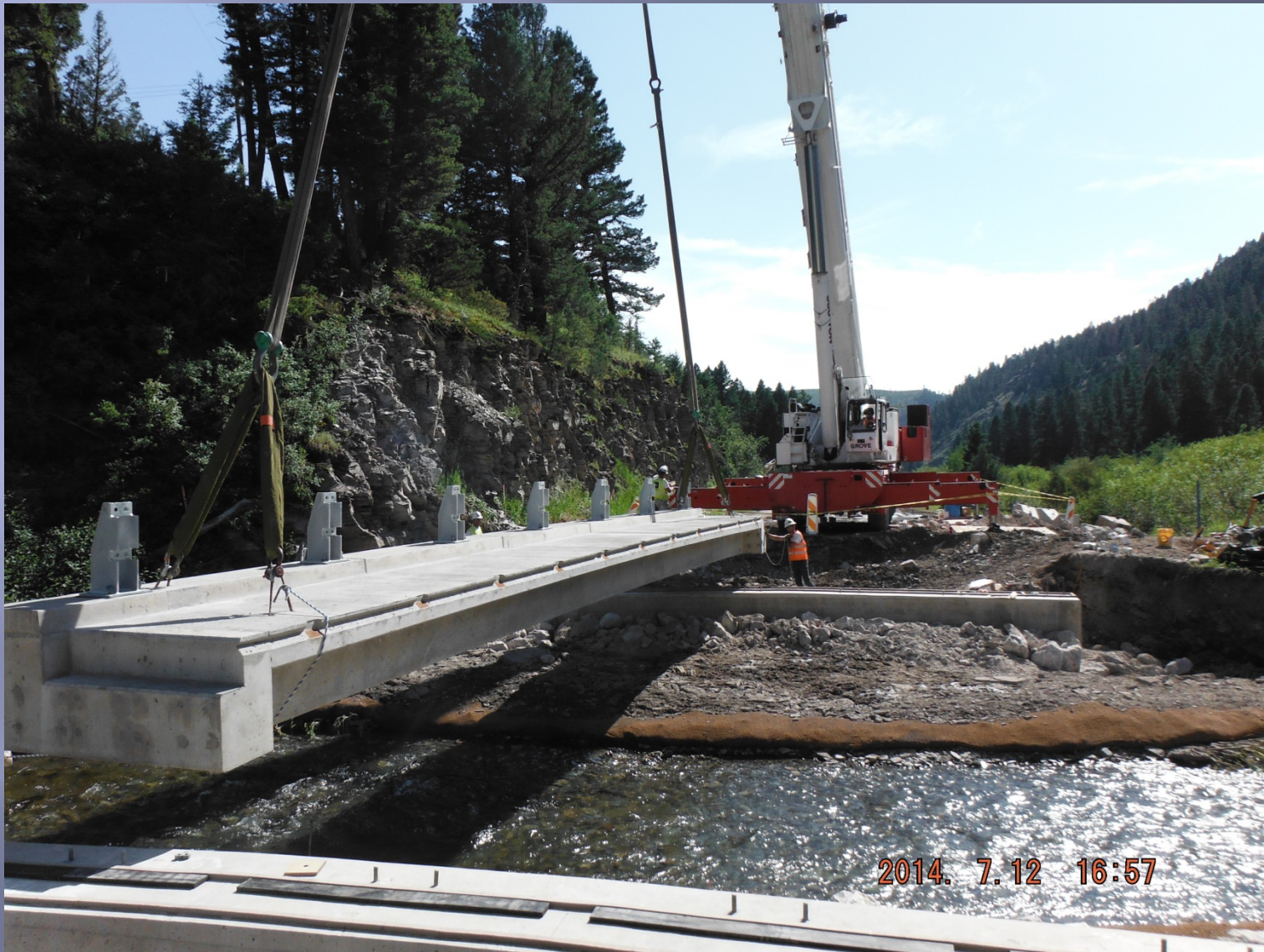
Prefabricated Bridge Element System
