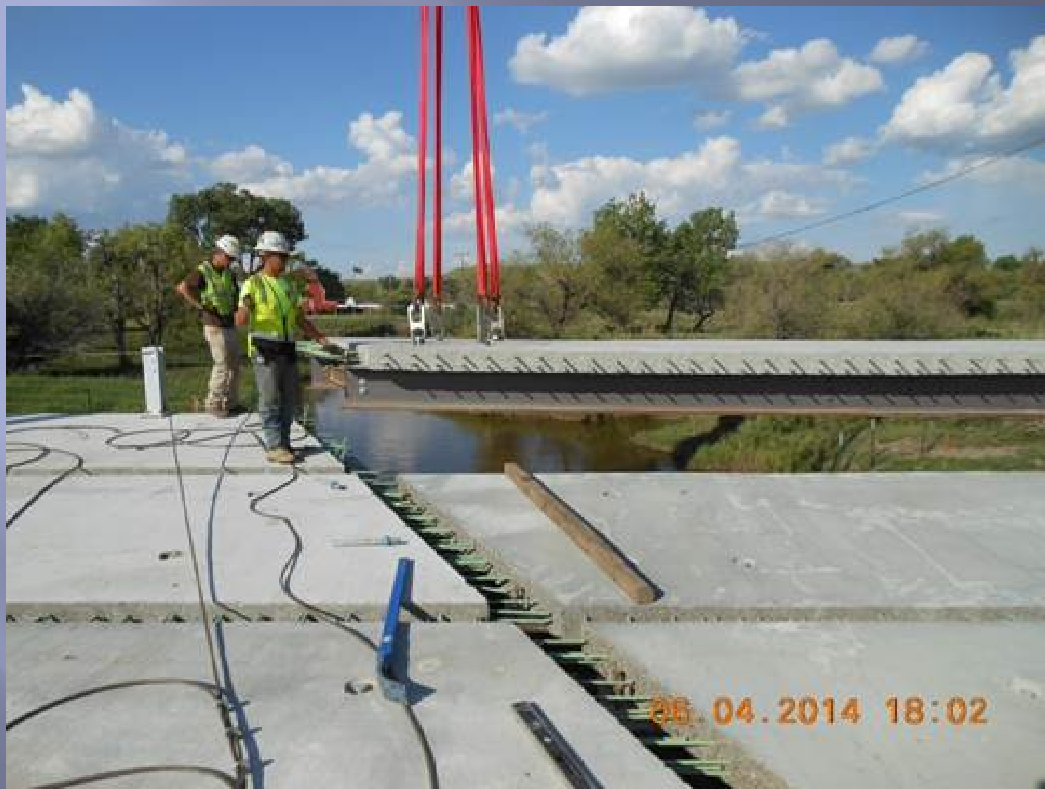
Modular Steel I-Girders with Integral Concrete Deck and CIP Closure Pours
