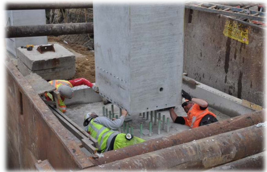
Column erection
