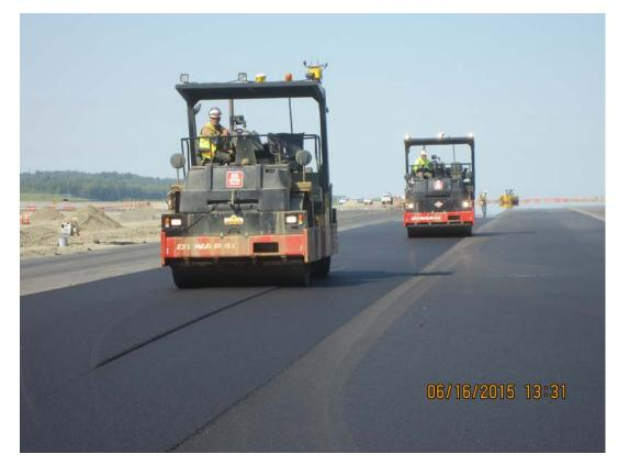
• Effect of reduced compaction or higher air voids because of lower mat temperatures.
