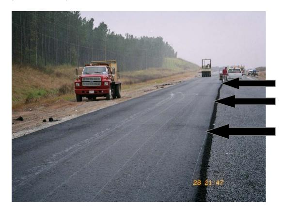
• Both sided longitudinal and centerline segregation result in thermal streaks; IR can identify these areas.
