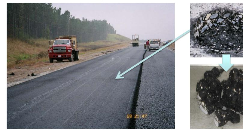
• Truck to truck segregation results in cold spots; IR can accurately identify these areas.
