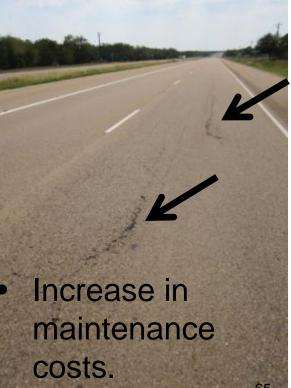
Thermal streaks; areas with increased potential for longitudinal cracking.
