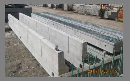
Precast Beams with Integral Bridge Rail
