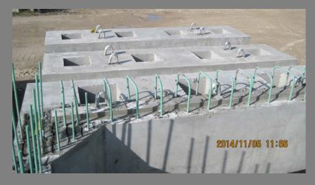
Precast Abutments and Pile Cap
