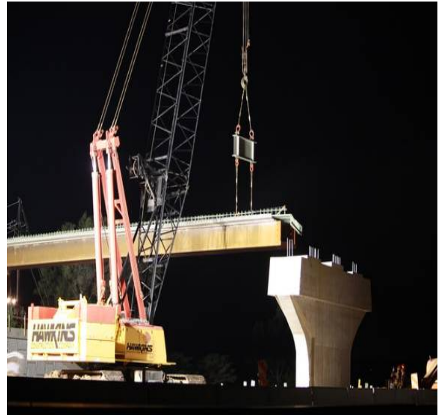
First Girder Approaching Pier
