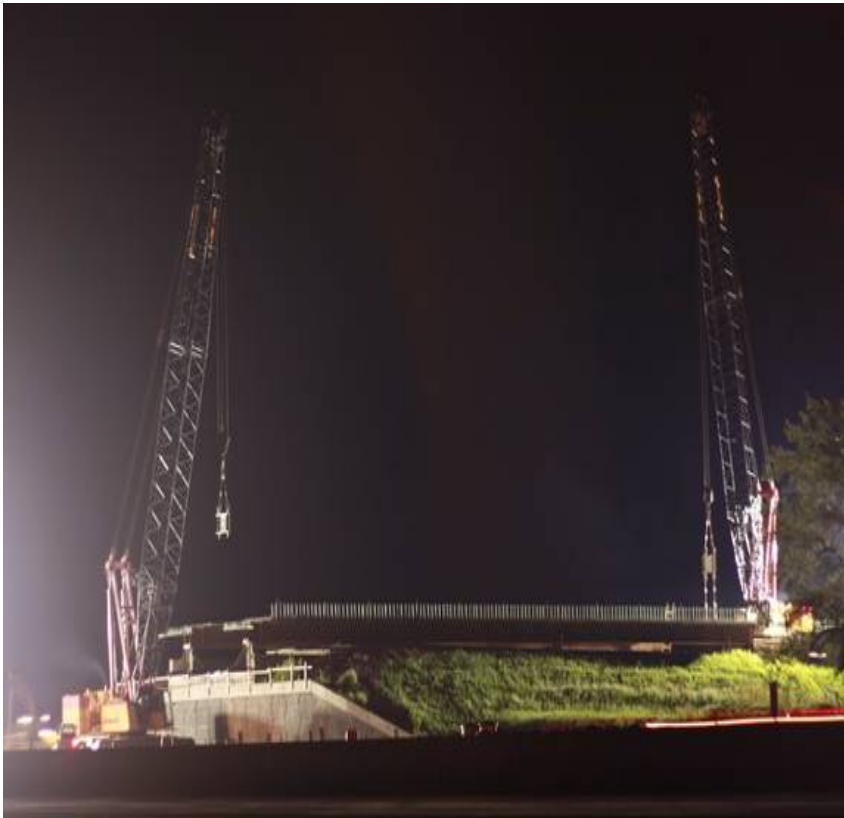
Cranes in Position for First Lift
