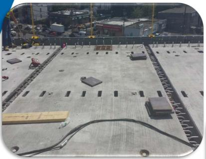
Exodermic Deck Panels – The design also incorporated Precast Exodermic Deck Panels at the eastern end and in/around the Broadway Ramp where weight was a concern due to planned widening
