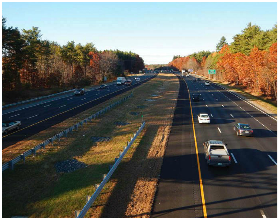
Completed view of U.S. 3 following all pavement preservation applications
