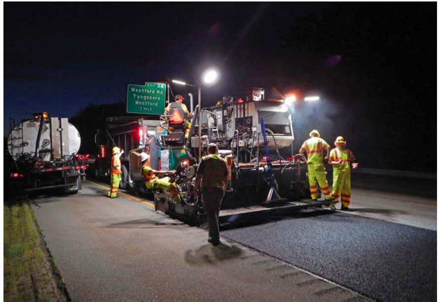
Spray paver places ultrathin bonded overlay treatment
