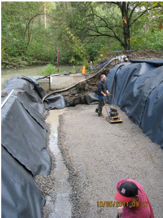
Backfilling Geotextile
