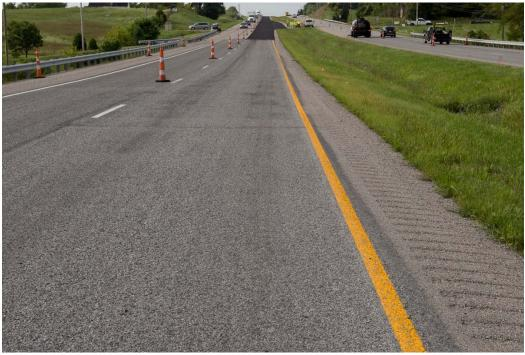
Figure 3. Chip Surface before Cape Seal Microsurface Placement (source: Strawser Construction, Inc.)
