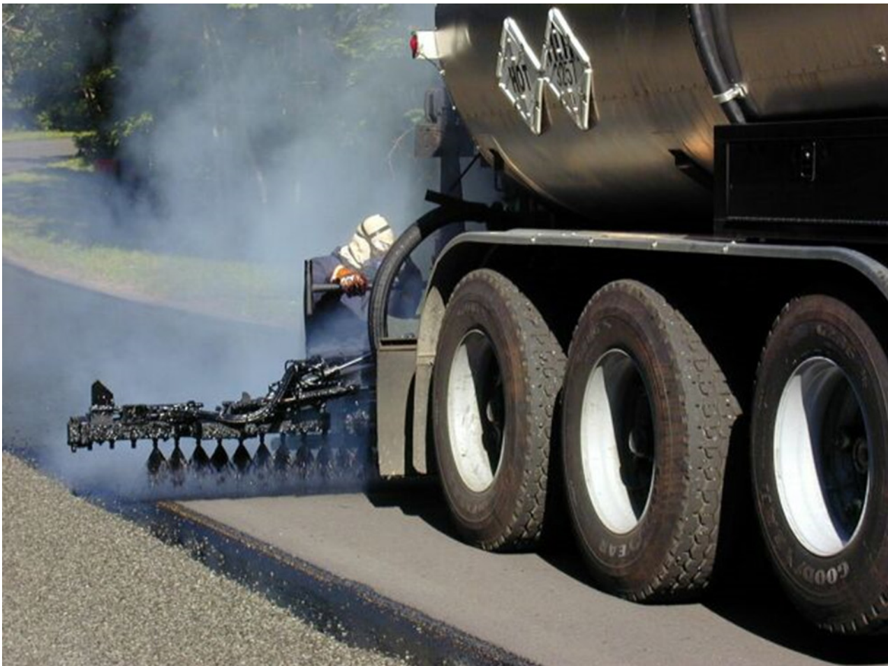
Figure 5. Rubber-Modified, Hot-Applied Binder Distributed as Part of the ARCS Treatment (source: RIDOT)
