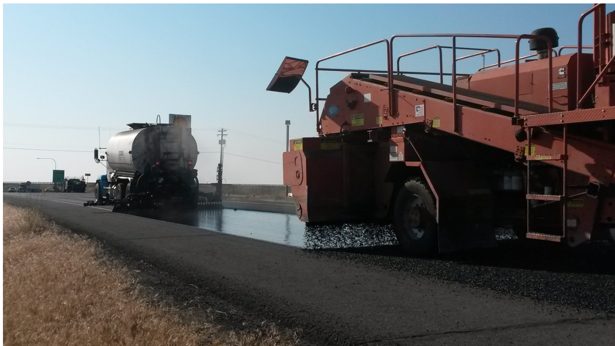
Figure 2. Pre-coated chips are dropped onto the asphalt cement to provide the wearing surface.
