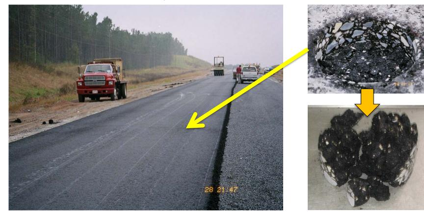
Truck to truck segregation results in cold spots; IR can accurately identify these areas.
