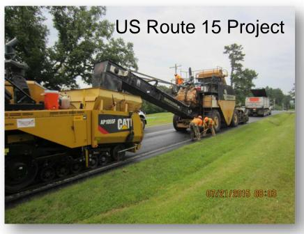
Mixture placed with Caterpillar paver. MTV used on the US Route 15 project.
